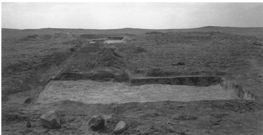
2. View along the pylon foundation from the north.
